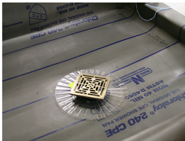
Installed in a full mortar bed method shower with Chloraloy® shower pan liner.
